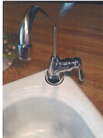
Under-the-sink POU treatment system with dedicated dispenser on kitchen sink
